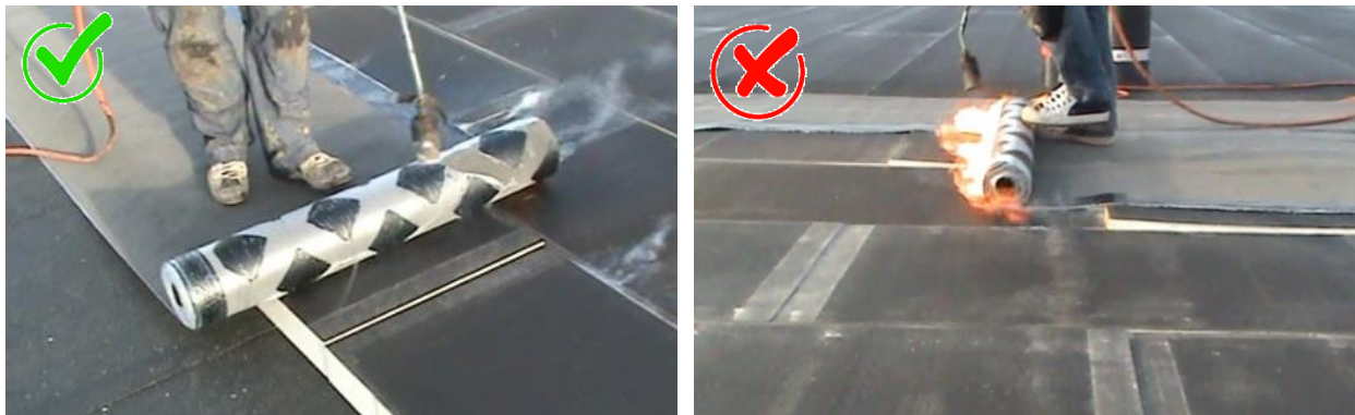
Figure 8: Torched application on a PIR insulation board to indicate good practice (left: partially adhered base layer with torching on roll; right: torching on insulation board)
