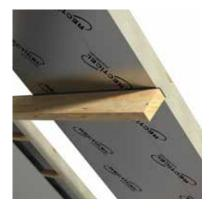
Installation L-Ments® are installed perpendicular on to the purlin structure of the pitched roof.
