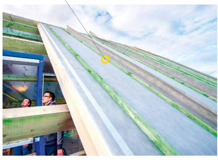
The Rectitape<sup>®</sup> insulation tape means it's easy to make joins airtight.
