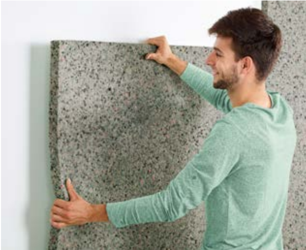
Positioning of the panels before applying glue.
